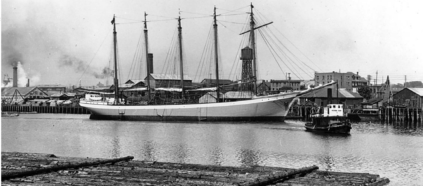
The 240' x 44' five-masted auxiliary schooner (twin Bolinder semi-diesels) LAUREL WHALEN, a Mabel Brown-class lumber freighter, is shown here in 1917 in the Upper Harbour at Victoria BC. She was launched that year by Cameron-Genoa Mills Shipbuilders Ltd.
